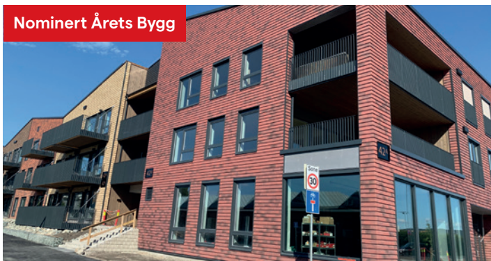
Gartnersletta – Powerhouse Lade
